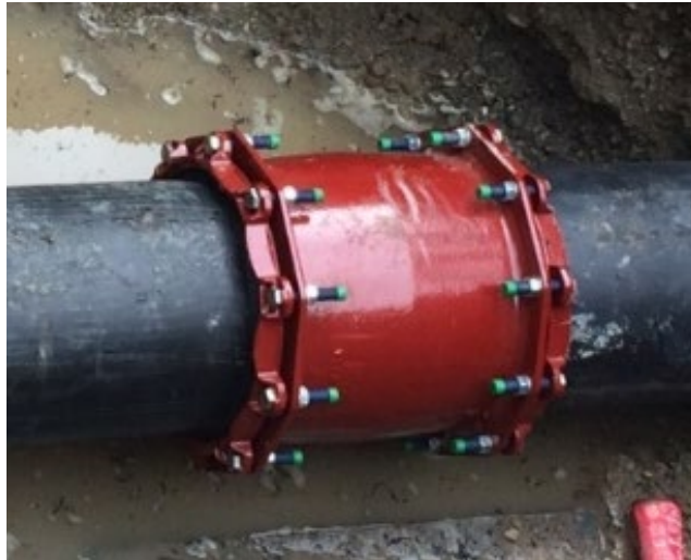
Figure 1 - Example of a bolt tightening design of fitting installed on PE pipe (Image courtesy of Georg Fischer Piping Systems)
